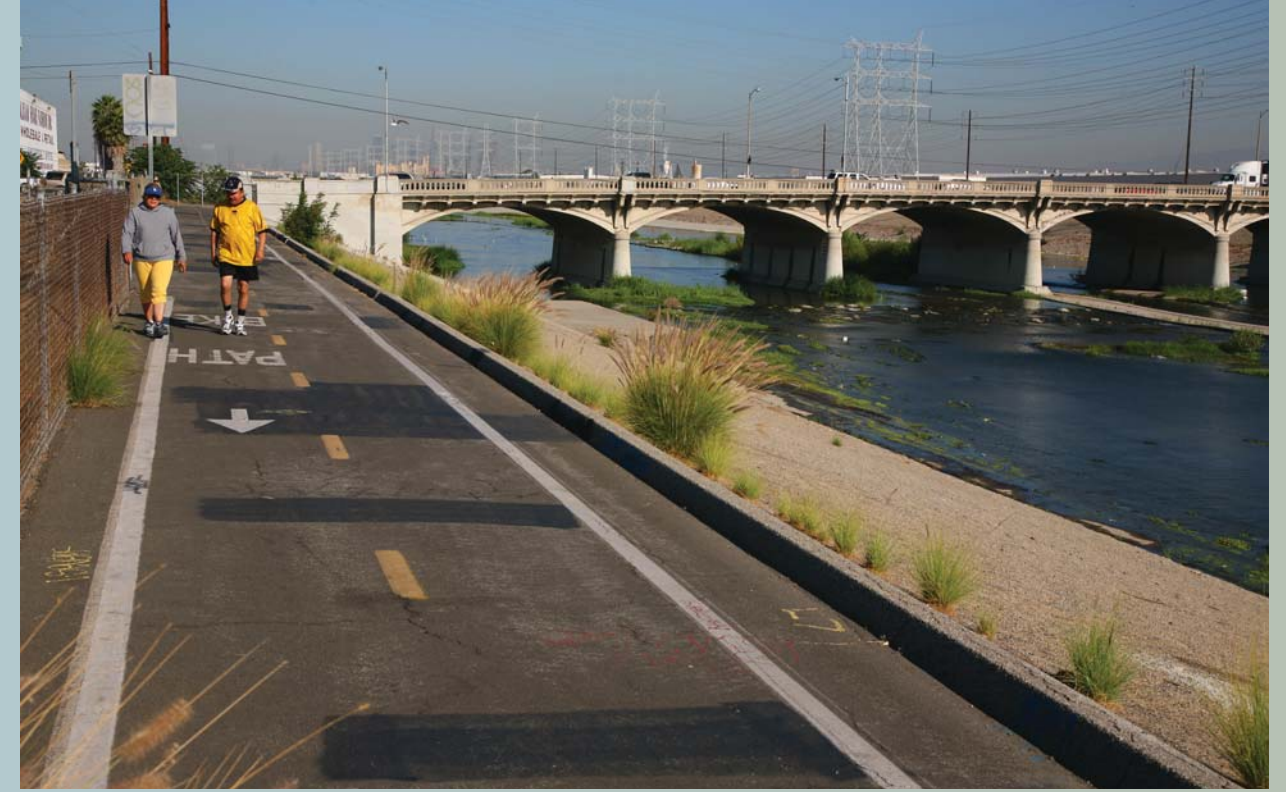
Reducing stormwater pollution and protecting the LA River is a major goal for Vernon
