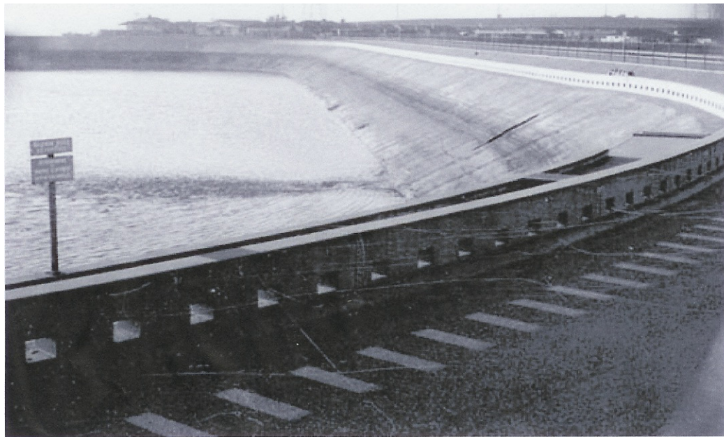
Baldwin Hills Dam - Dark spot in upper right hand quadrant shows the beginning of the break in the dam.
