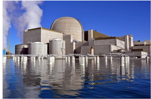
Figure 49. Palo Verde Nuclear Station
