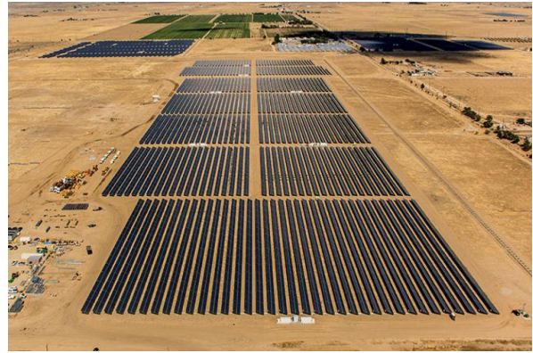
Figure 53. Antelope DSR 1 Solar PV Facility
