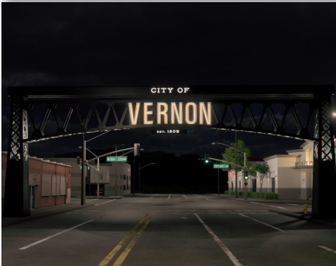
Vernon's Gateway Arch is being installed at the intersection of Santa Fe and 25th
