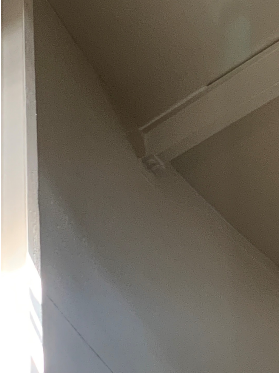
Figure 4: Rafter to shell connection
