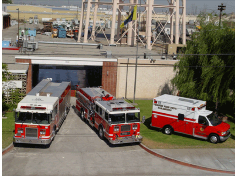
Vernon Fire Station #3
